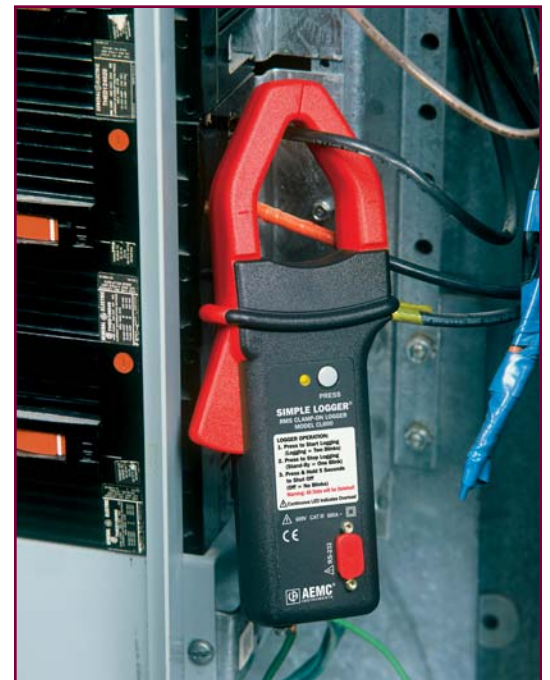
Model CL600 recording current draw on a VSD
