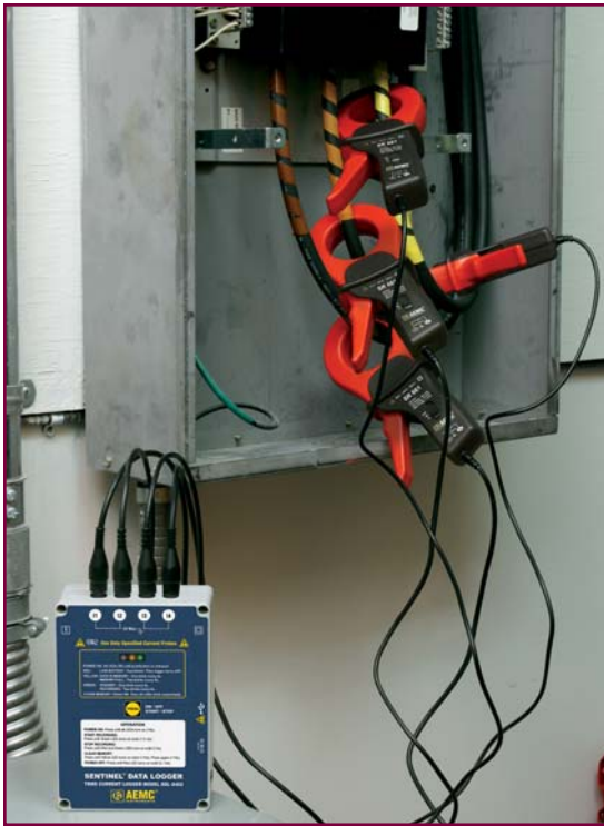
Model SDL A402 recording phase and neutral currents on a feeder.
